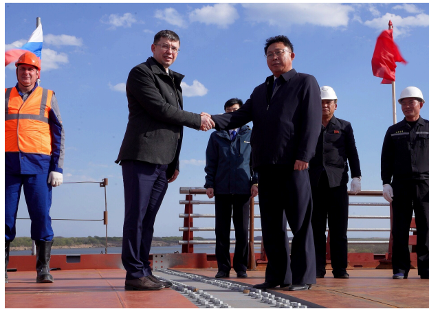
A handshake marks the joining of the spans of the Yakov Novichenko road bridge over the Tumen River between Russia and North Korea, then under construction, 21 April 2026.
